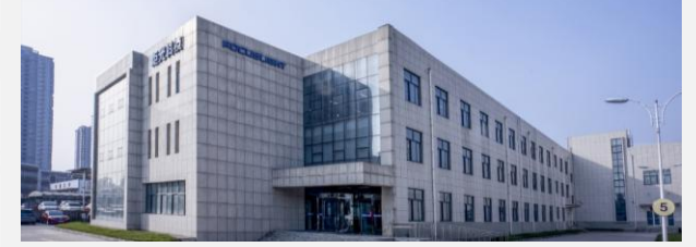
Xi'an, China Focuslight HQ, Operation Center
